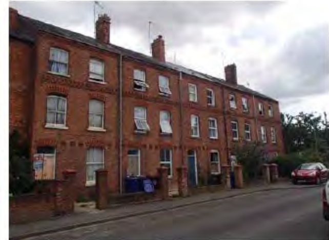
Narrow fronted 3 storey terrace, Banbury
