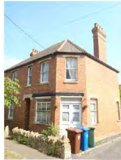
Cutting off edge to address corner, Islip
